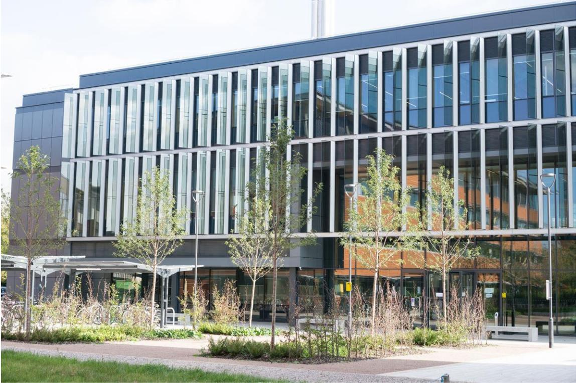
Dugan added, *“This is also the first project that has been designed and fitted with thermochromic glass fins externally. The Suntuitive Dynamic Glass on the facade tints as temperatures warm and intuitively allows daylight in while limiting the UV and glare penetrating the building. This gives the structure the ability to maintain best temperature and comfort.”*
