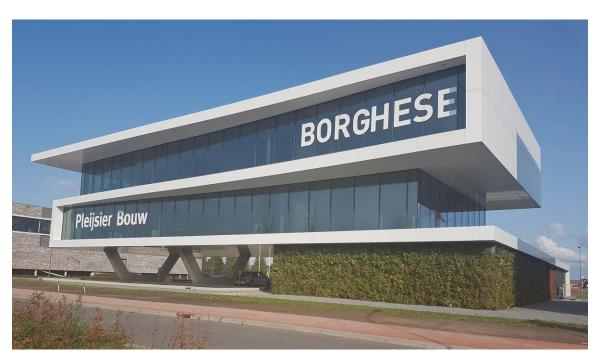
"The building was designed to be open, with a lot of glass and without too many walls. To create an open structure, we chose not to use any sunscreens or other objects that will stand in the way of such a design. Therefore, we selected Suntuitive glass. The transparency and open structure is not only for the design of the building but also the appearance that both companies portray," said Sep de Bruin of Pleijsier Bouw.
